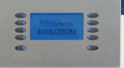
The Evolution Control System installed at The O2 operates over 3000 lighting circuits with individual control of hospitality rooms, concession areas and general circulation space as well as the main Arena itself. Localised operation is provided by control plates while a graphics based PC software provides control of the whole venue including the ability to drill down to individual areas and obtain status feedback.
