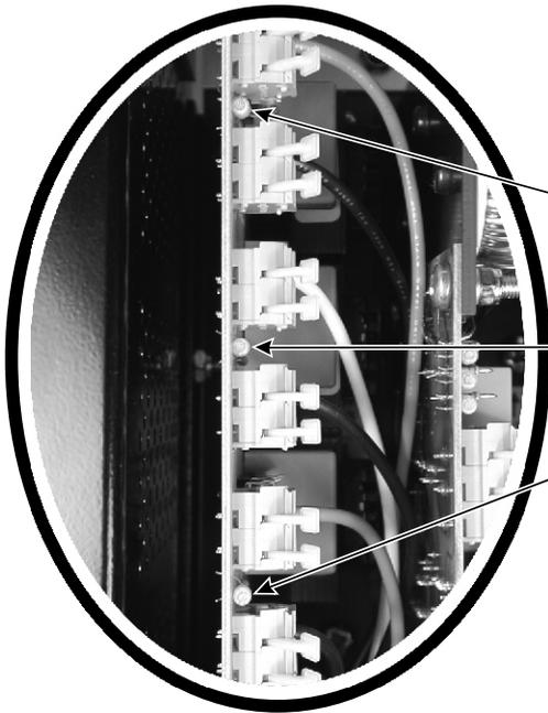
The three neons shown indicate when the phase input is live.
